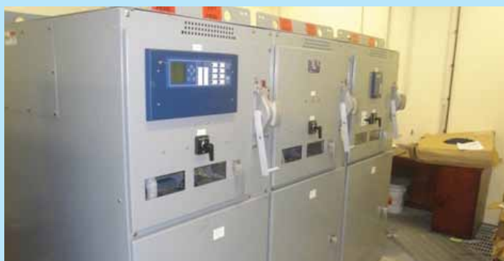
Switchgear installed in Generation Building at SGU.
