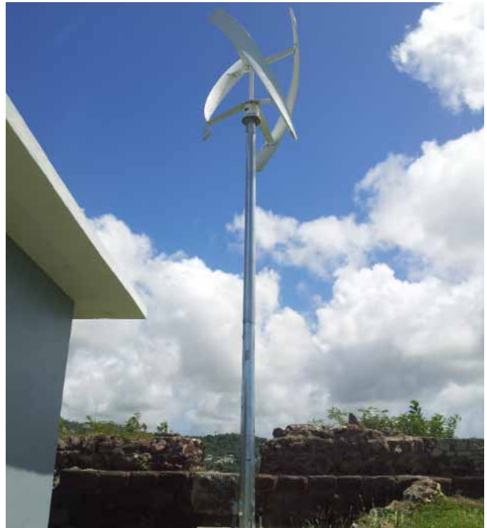
Vertical axis turbine and solar panels - Renewable Energy Demonstration Project at Fort Frederick.
