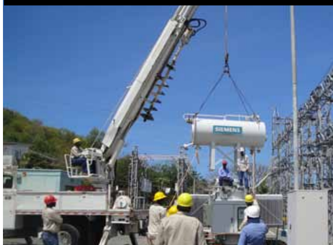
Installing Substation Transformer.
