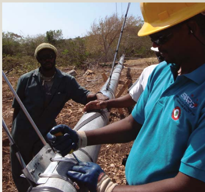
Installing wind measuring equipment.
